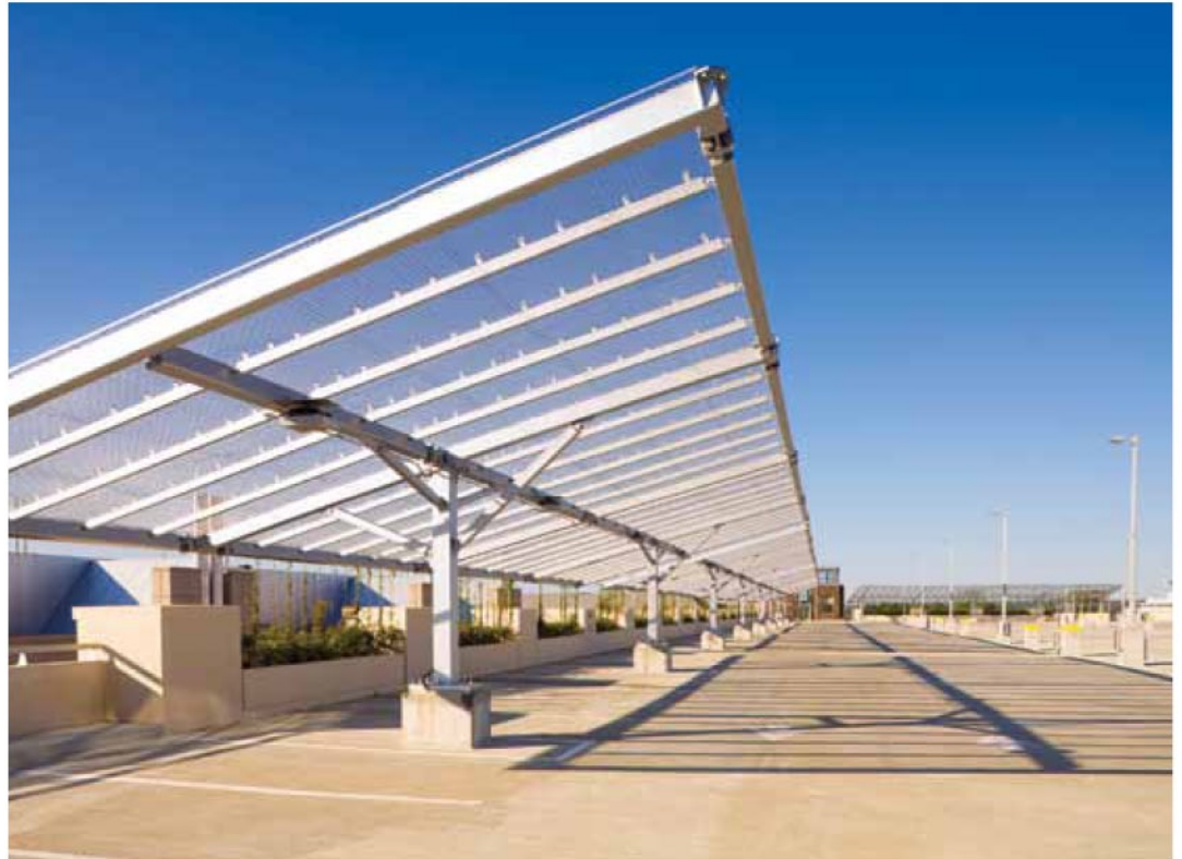
Solar carports can generate electricity and reduce heat island effect.
